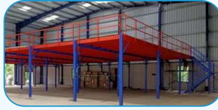
Modular Mezzanine Floor
