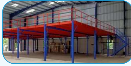
Modular Mezzanine Floor
