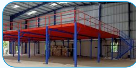
Modular Mezzanine Floor
