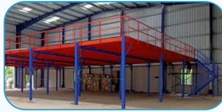
Modular Mezzanine Floor
