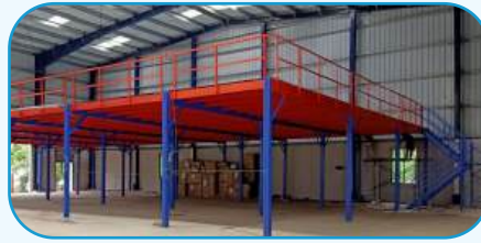
Modular Mezzanine Floor
