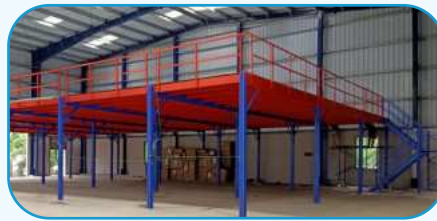
Modular Mezzanine Floor
