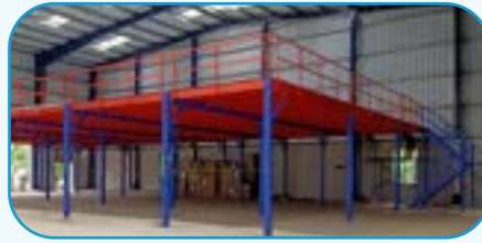
Modular Mezzanine Floor
