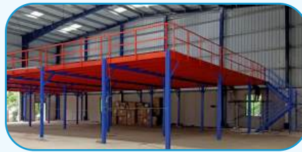
Modular Mezzanine Floor
