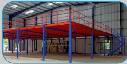
Modular Mezzanine Floor
