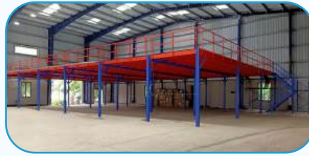
Modular Mezzanine Floor
