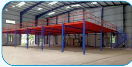
Modular Mezzanine Floor
