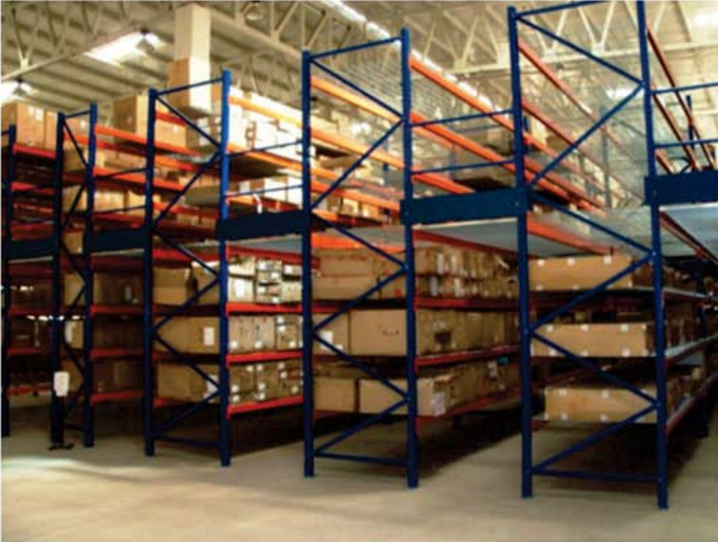
Long Span with Multi-tier Racking Systems
