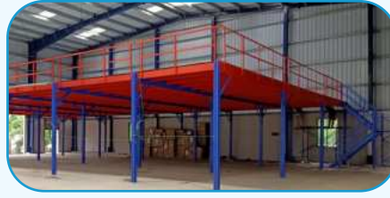
Modular Mezzanine Floor
